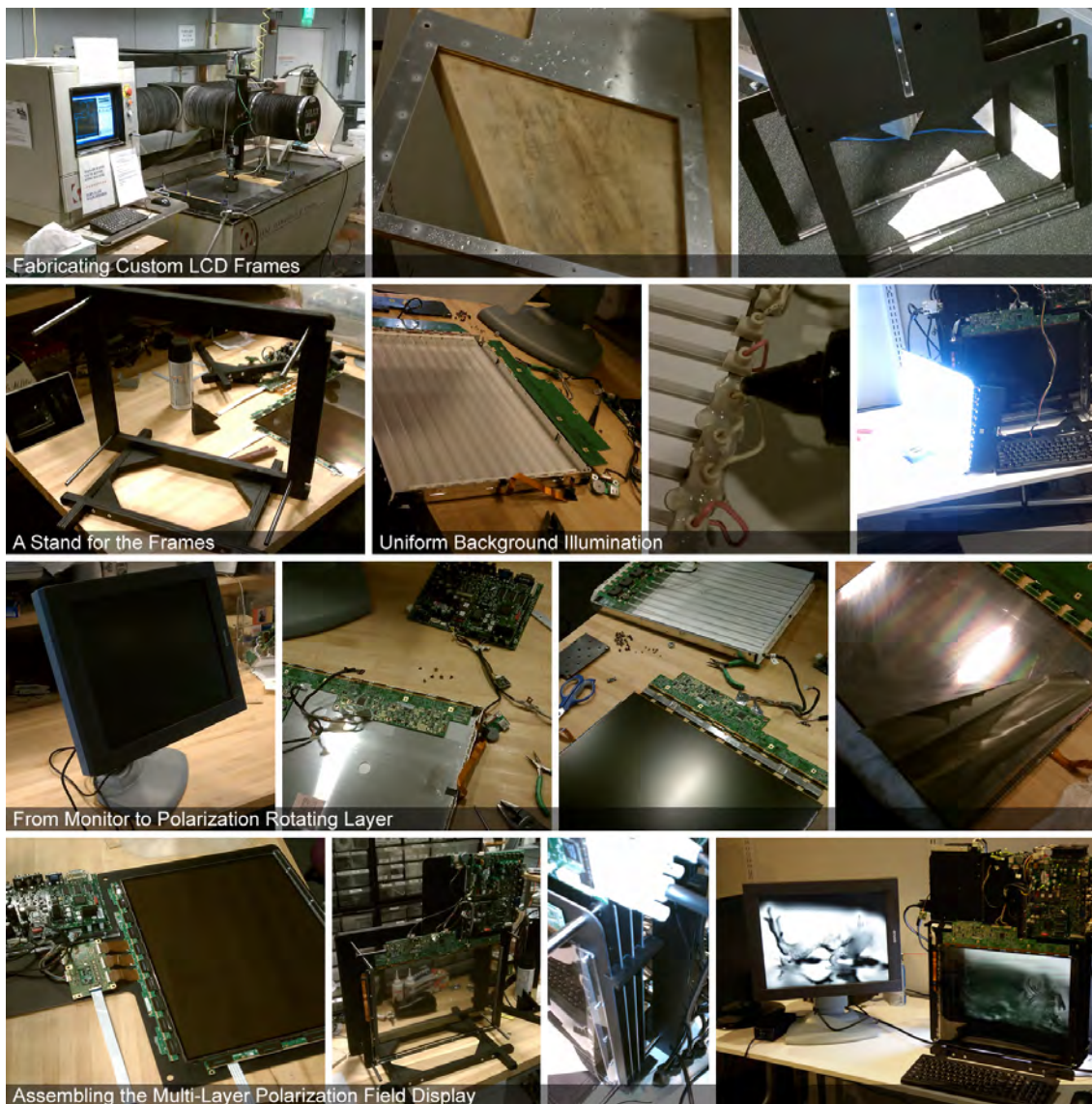
Figure S.1: Photographic documentation of the prototype construction. Four monochrome, off-the-shelf medical LCDs were modified. Polarizing films were removed and electronics repositioned so the panels could be mounted on custom-fabricated frames. The layers are separated by acrylic spacers and illuminated by a uniform backlight.
